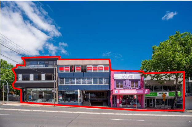
Picture 1: Pacific Highway frontage
